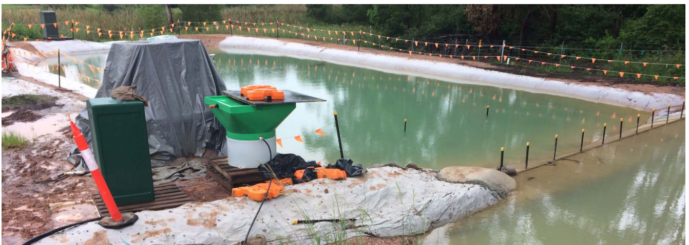
Temporary HES basin (Highway Construction)
